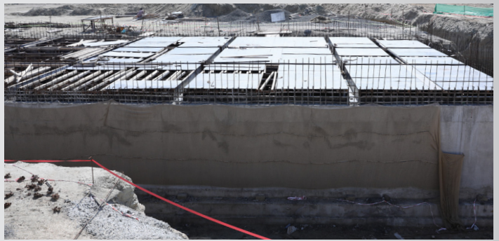
250,000 Gallons Underground Water Tank
